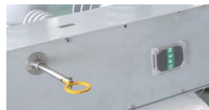
Lockout handle-pulled (open position)
